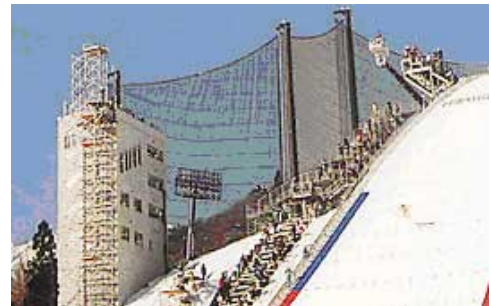
Windbreaker/snow protection net used for the Hakuba Ski Jump Stadium at the Nagano Olympics.
